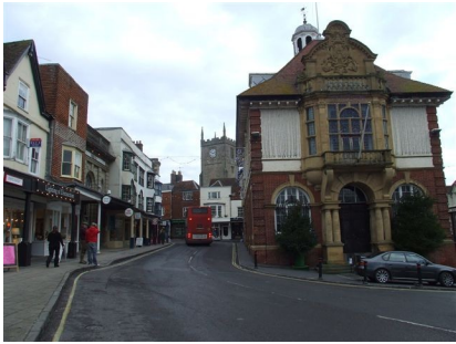
Marlborough Town Hall
